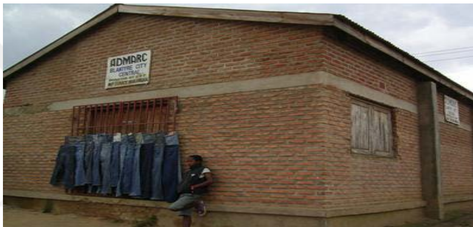
Figure 8 Showing ADMARC depot built with CDF funds by MP Makanagala, Blantyre Central
