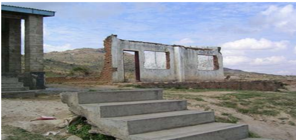
Figure 9 showing CDF-built school block at Matope, Ndirande, Blantyre (2007)
