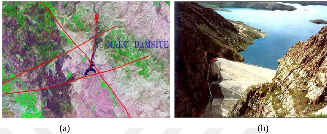
Figure 5.4 : (a) Satellite image of the Maku Dam site and the existing faults. (b) An oblique view of the Maku Dam
