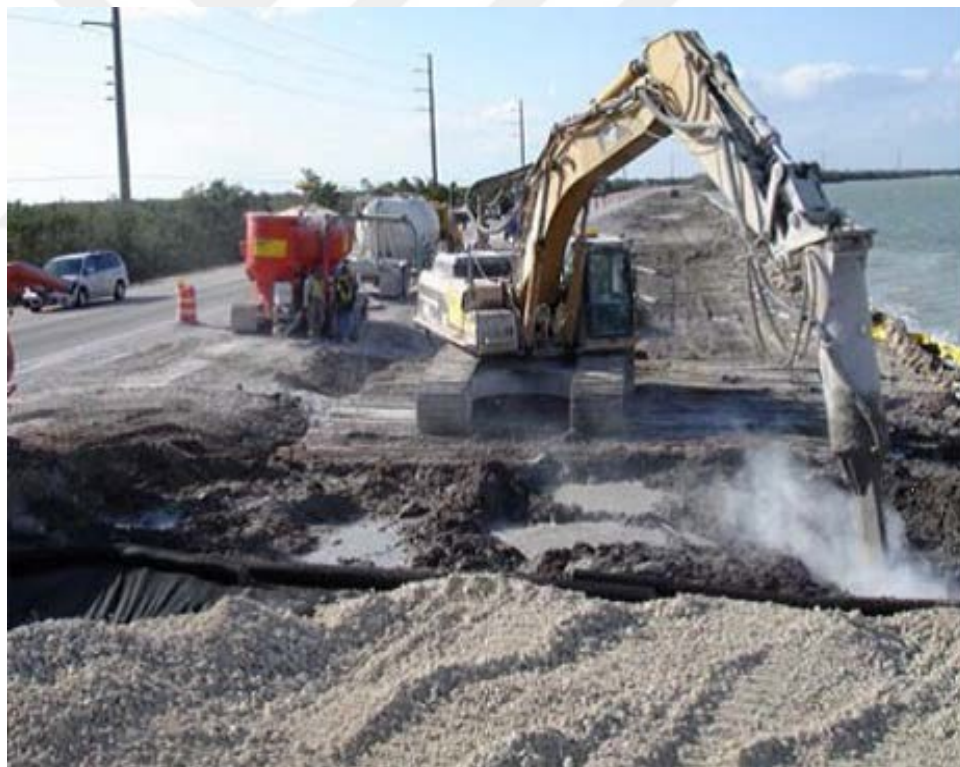
Figure 2.19 : Dry mass soil mixing to strengthen soft soils beneath a planned roadway expansion at U.S. Highway 1, Key Largo, Florida (Hayward Baker Inc).
