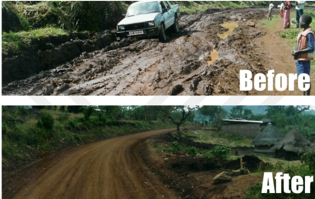
Figure 2.21 : Effect of CBR Plus before and after of the stabilization (International CON-AID Ltd.).
