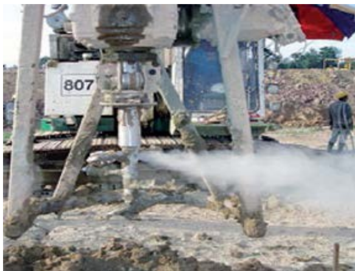
Figure 2.14 : Injection of dry binder into the soil from the mixing tool (Keller Inc.).
