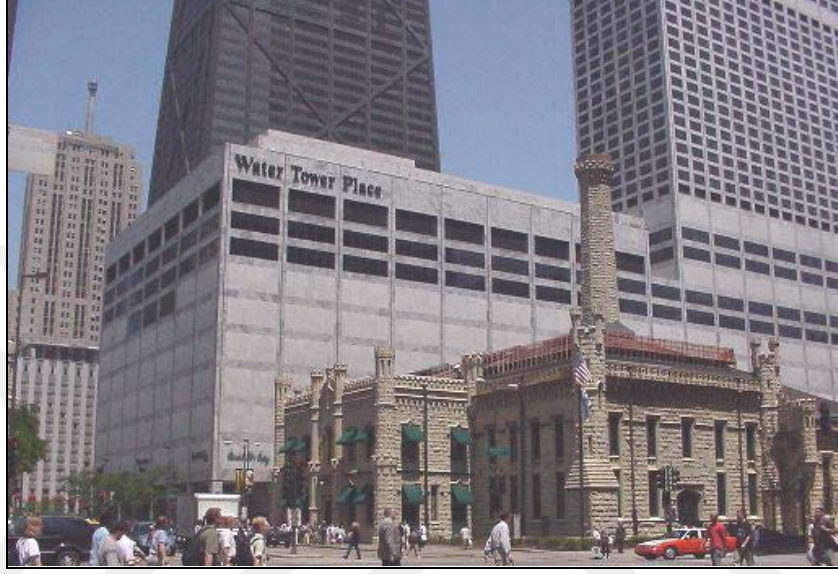
Şekil 3.10 : Water Tower Place, Chicago (Url-7).
