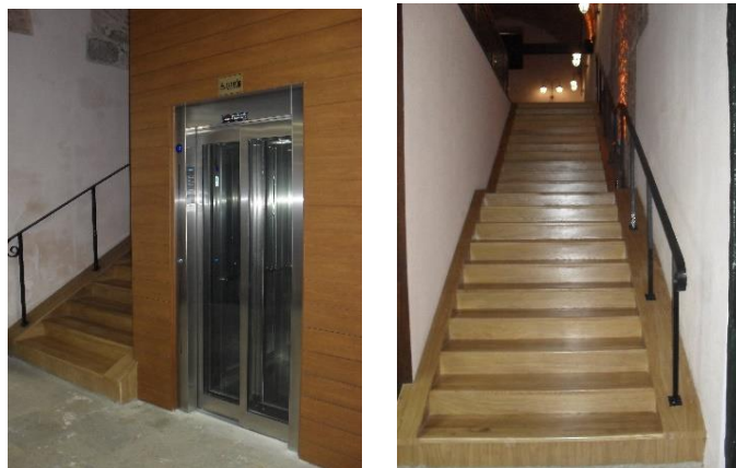
Figure 4.16 (a) Lifts made inside the 'Sandal Bedesten', (b) Details of the built stairs created in the side of an old gate, taken by author on 18th of October 2016.
