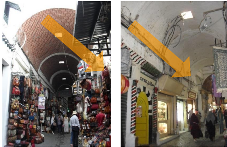
Figure 3.29 (a) Left: entrance of “Al-Trouk” bazaar, (b) right: electricity and air cooling cables in the bazaar’s roofs, developed by author taken on 20th of July 2016
