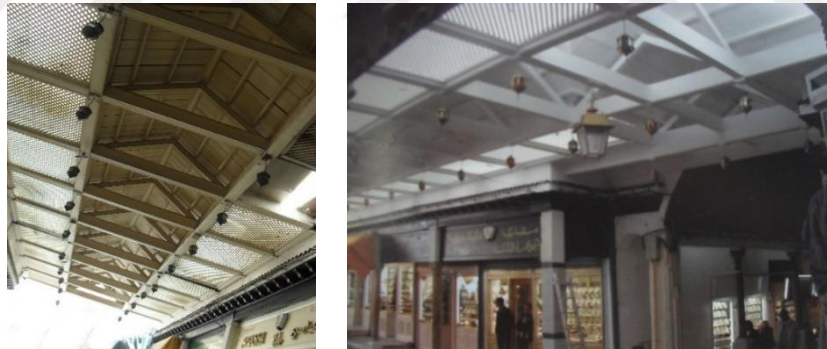
Figure 3.35 (a) Restored roof of one street from “Al-berka” bazaar, (b) Newly restored roofs, (a) provided by author on 20 th of July 2016; (b) [45]
