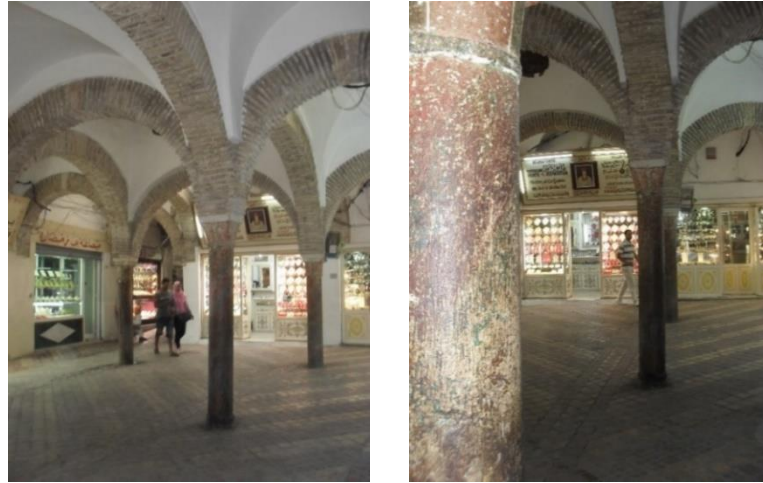
Figure 3.34 (a) Central area of the covered bazaar, (b) Ropes marks in columns, provided by author on 20th of July 2016
