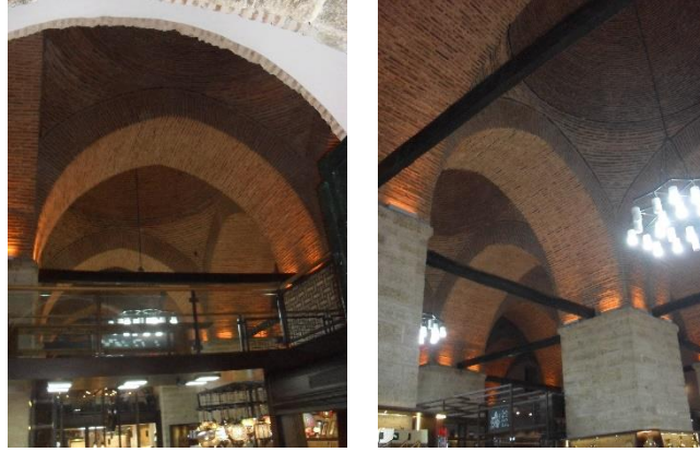
Figure 4.15 (a) View of the succession of cupolas, (b) Details of the building materials used, taken by author on 18th of October 2016
