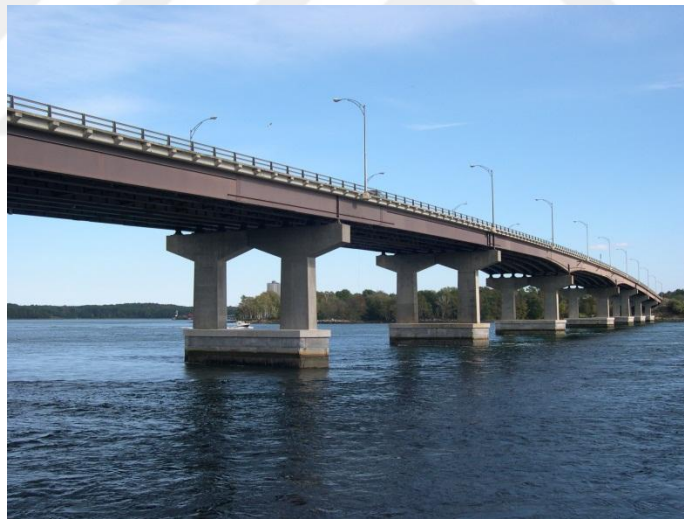
Figure 40. Girder Type Bridge
