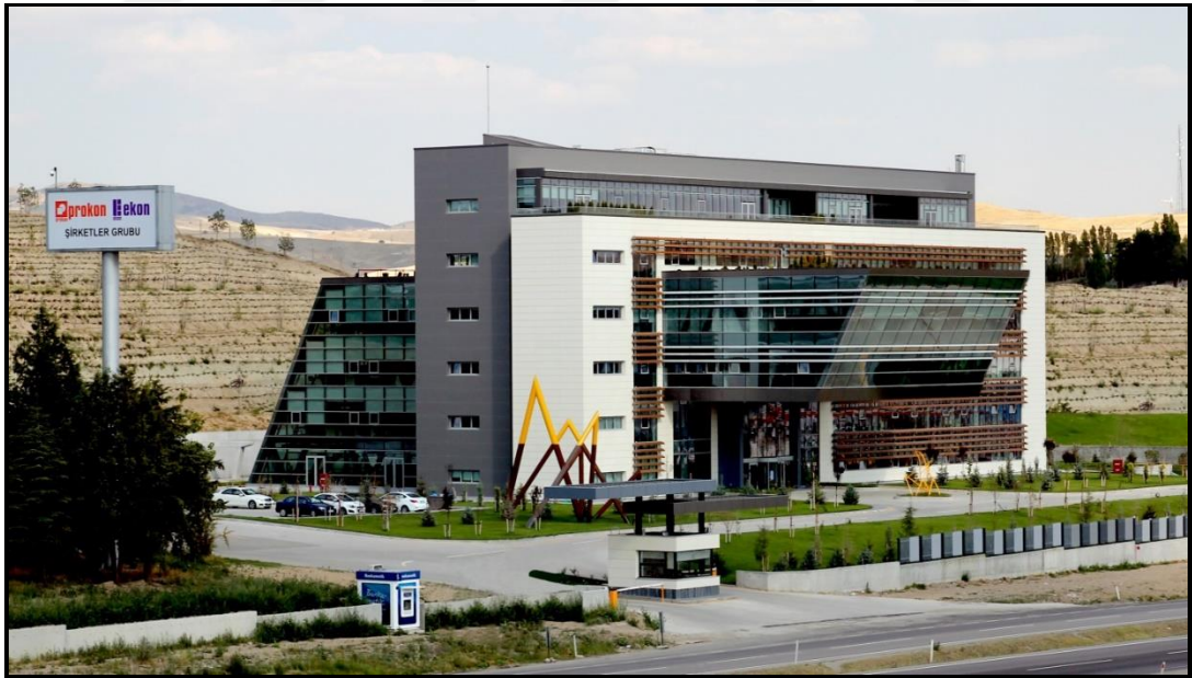
Figure 3.1. General view of Prokon-Ekon Office Building
