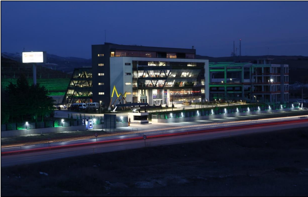
Figure 3.2. General view of Prokon-Ekon Office Building-II
