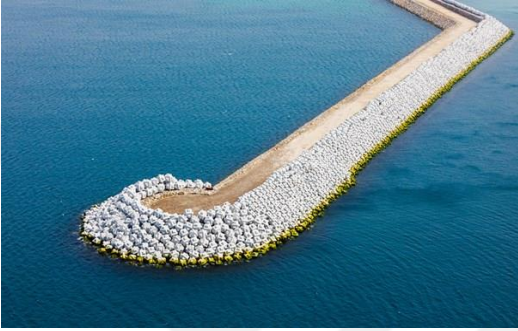
c) Beton bloklı dalgakıran (Cupipod), Port of Coruña, İspanya[9]
