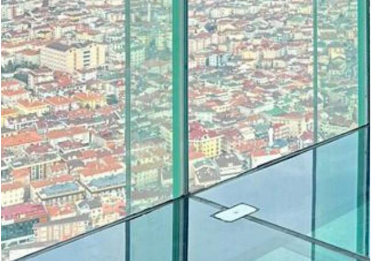
Picture 1.2 Laminated glass pane walls and floor slab
