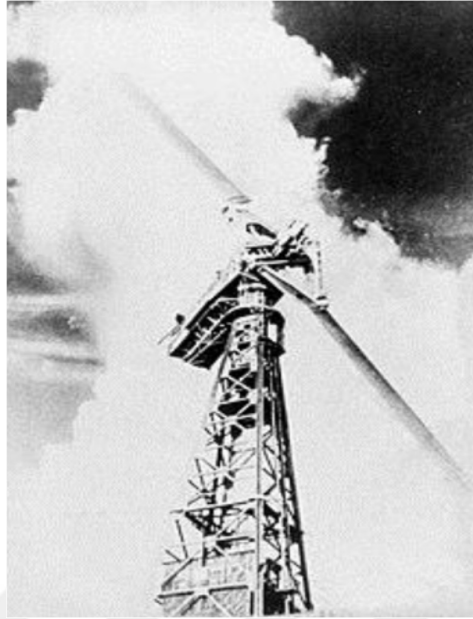
Figure 2.6. 1.250 MW capacitated Smith-Putnam wind turbine (Ragheb, 2010).
