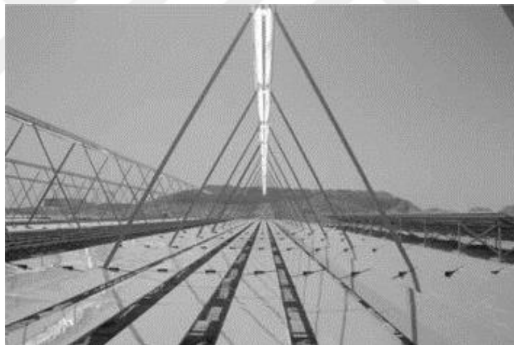
Figure 2.12. Linear Fresnel collecto [43].
