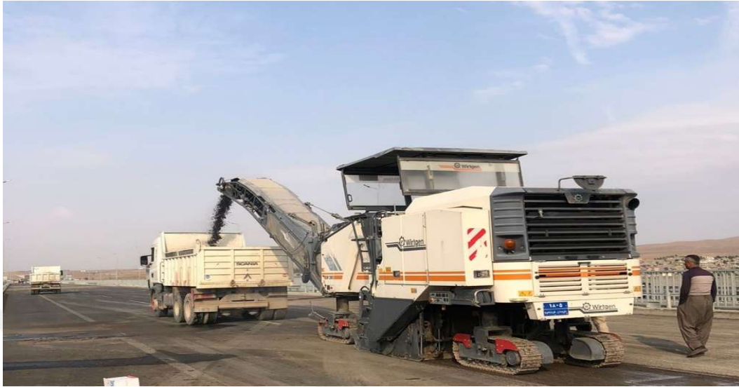
Figure 3.4. RAP Milling along Ankawa road in Erbil, Iraq
