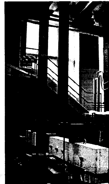
(b) Steel columns
