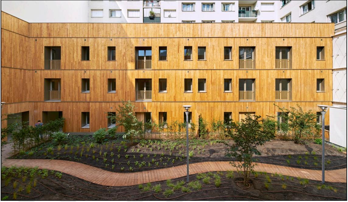
Şekil 3.12. 90 Housing And Office Avluya Bakan Cephe (URL-7)
