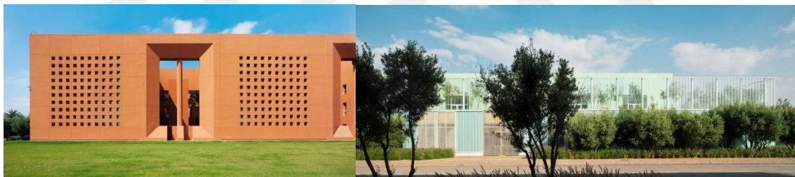
Image 50. University Polytechnic Mohammed VI, LEED silver certified buildings: Left: Learning building. Right: Pole Sport. Source: Recardobofill.com
