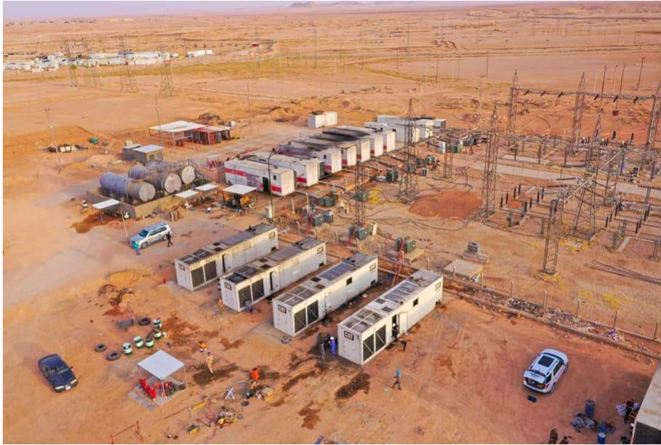
Figure 3.16. The power system plant in Rutba city.
