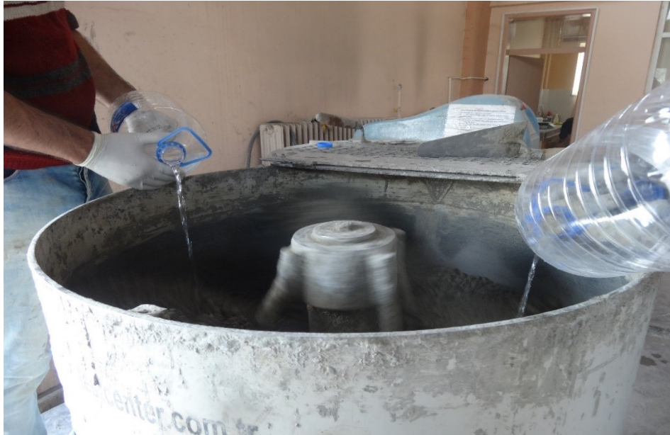
Figure 3.6 Wet mix (dry material, alkaline solution, sp, and water)
