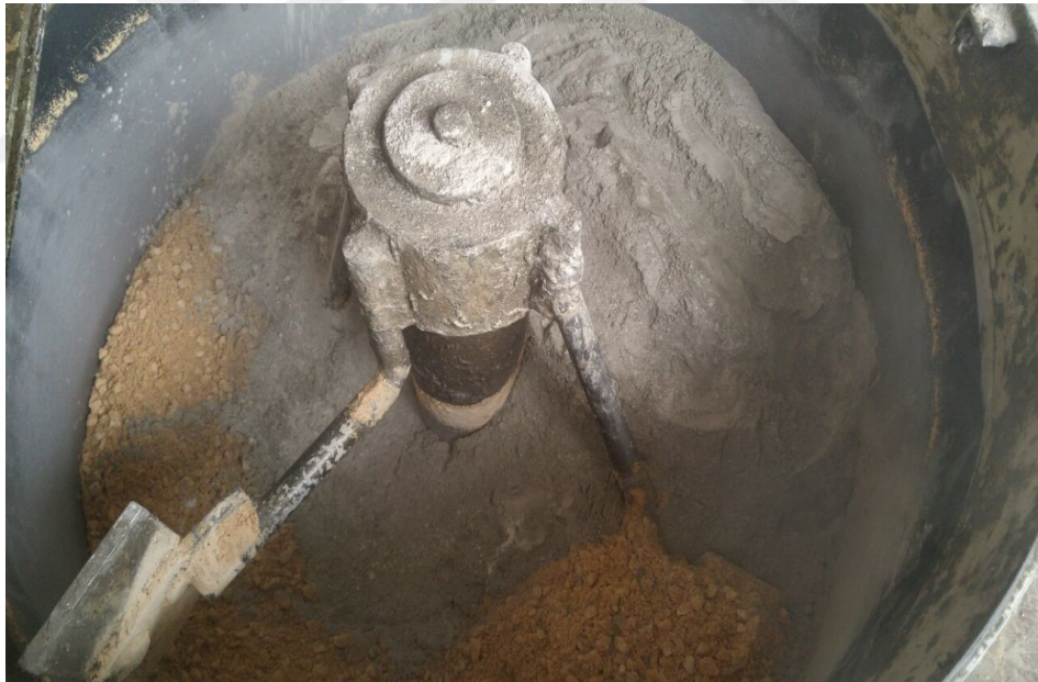
Figure 3.5 Dry material (binder, fine and coarse aggregate)
