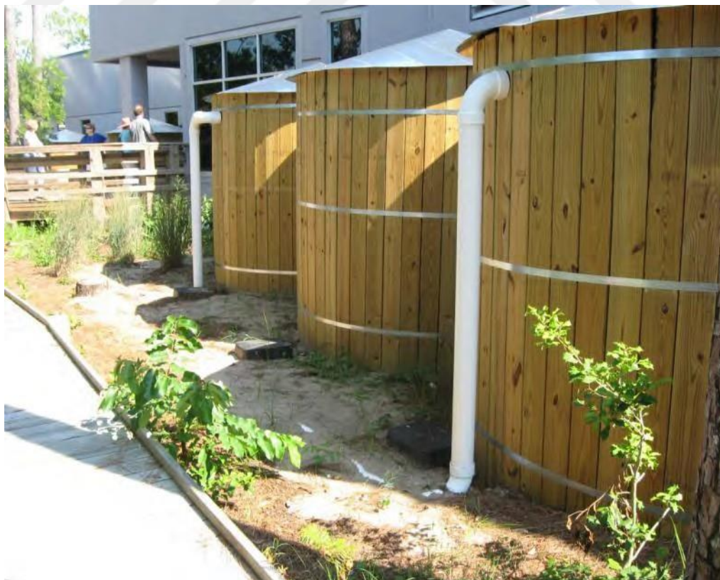
Figure 2.23 : Wood wrapped cistern.
