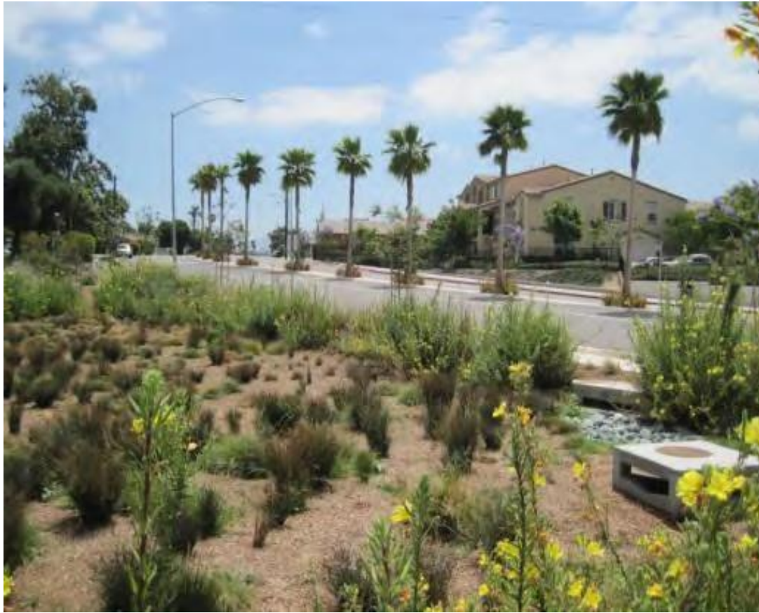
Figure 2.3 : Bio-retention area (San Diego, California).
