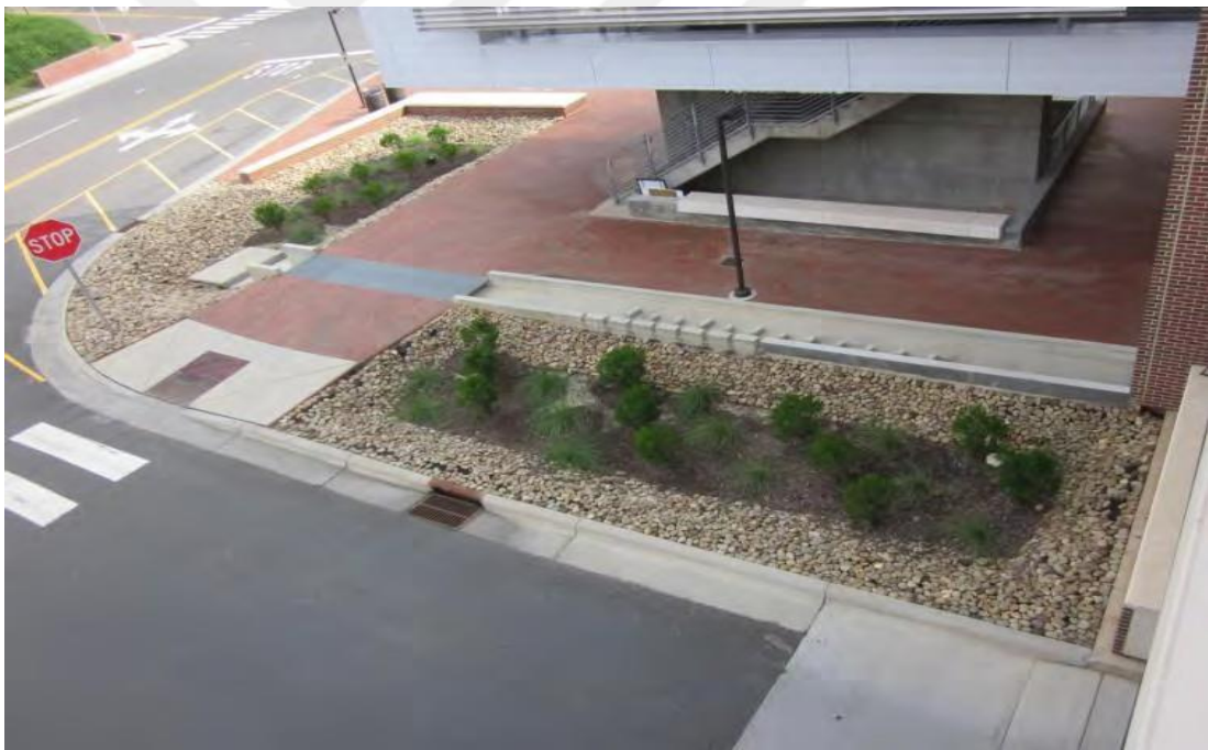
Figure 2.5 : Parallel bio-retention areas treat parking structure runoff conveyed by a concrete flume (North Carolina State University campus).
