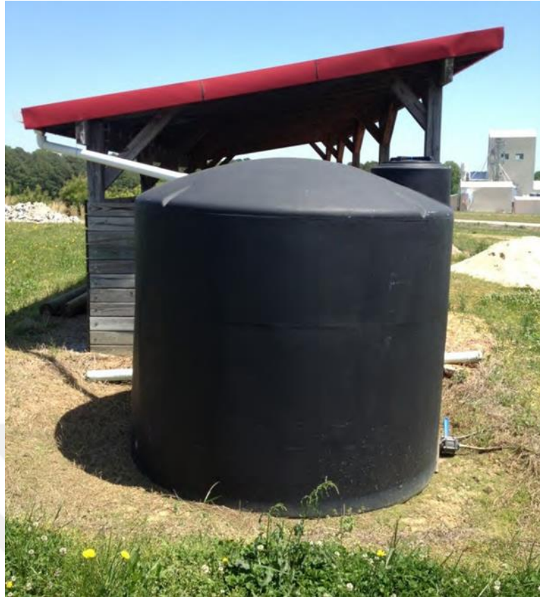
Figure 2.22 : Typical plastic cistern.
