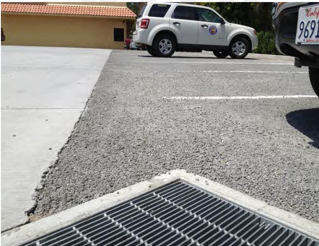
Figure 2.14 : Pervious concrete (San Diego, California).
