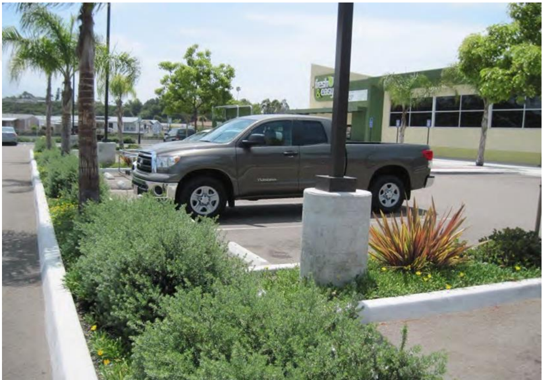
Figure 2.8 : Parking lot bio-retention swales (Oceanside, California).
