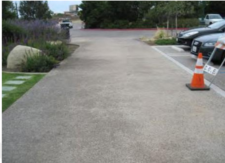
Figure 2.10 : Example of pervious concrete.
