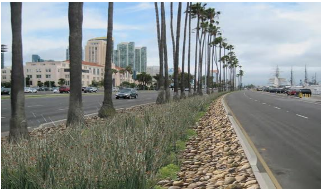
Figure 2.7 : Bio-retention swale in median (rendering).
