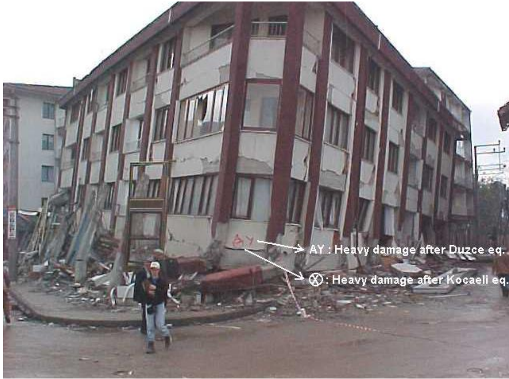
Figure 3.4. An example of a collapsed building during the Duzce earthquake that had already been damaged and tagged during the Kocaeli earthquake (Rathje et al. , 2006)
