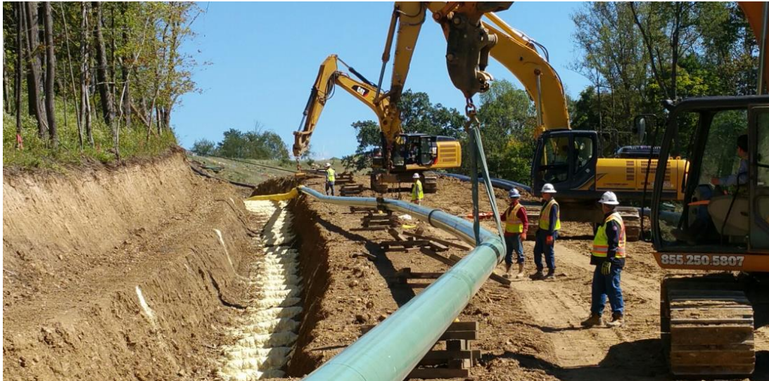
Figure 2.18 : Natural Gas Pipeline Construction
