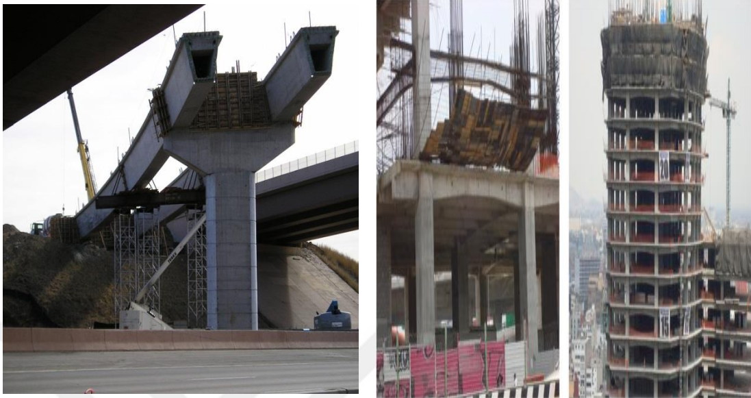
a. RCHBs in bridge
