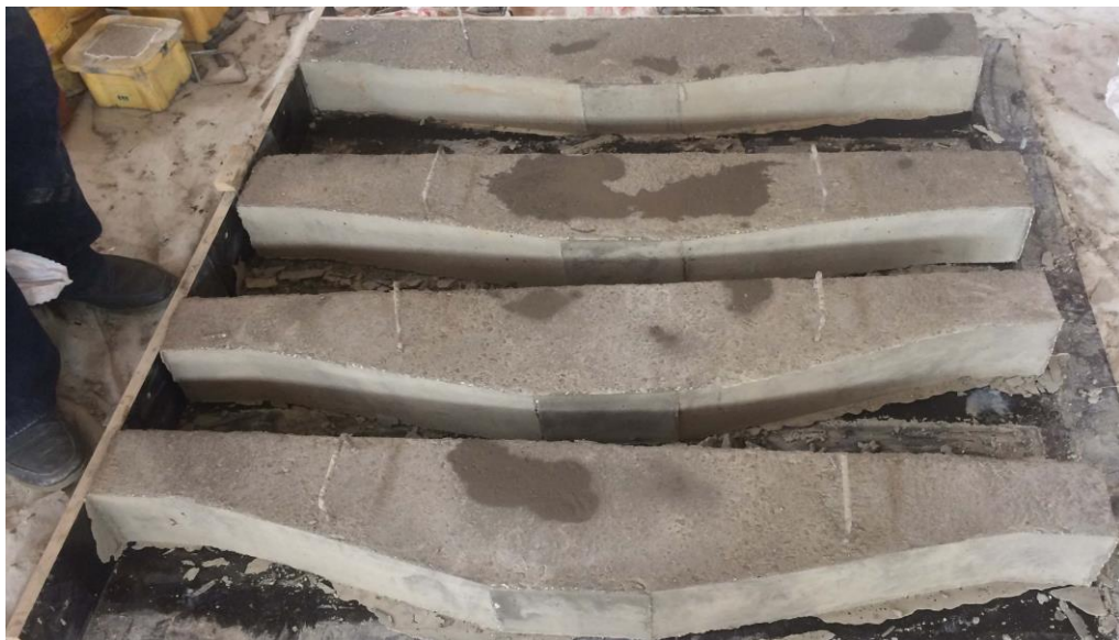
a. Removing formwork after casting
