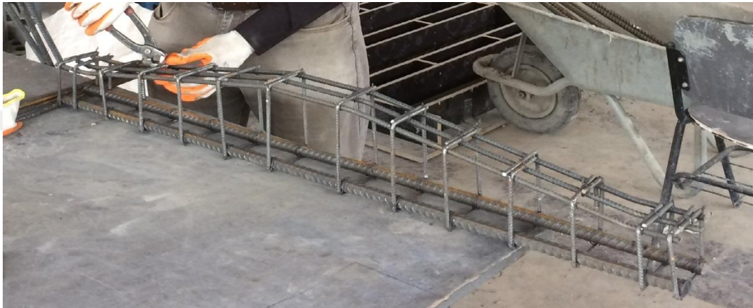
Figure 3.10 Reinforcement processing works
