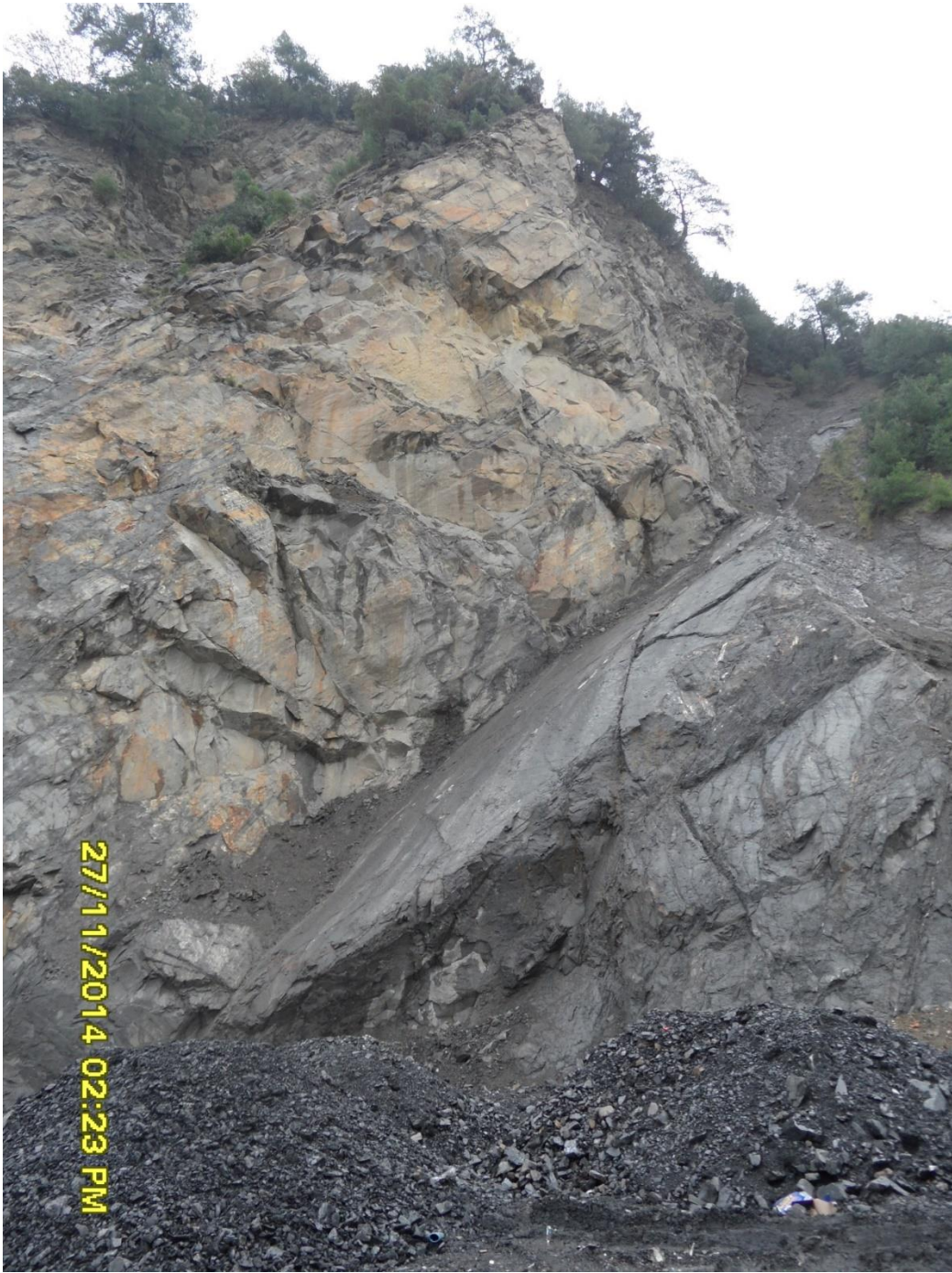
Figure 6. Rock mass structure at Kilimli, Zonguldak Aslankayası Tunnels site
