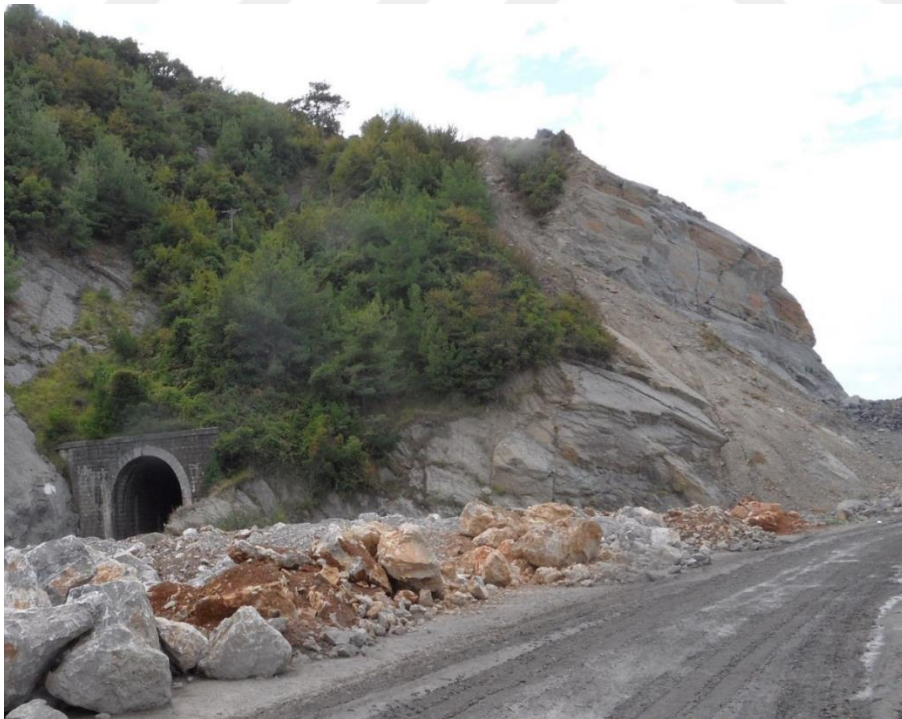
Figure 2. General view of the east portal of the tunnel and the surrounding rock
