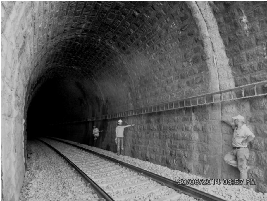
Figure 1. Inner view of the tunnel
