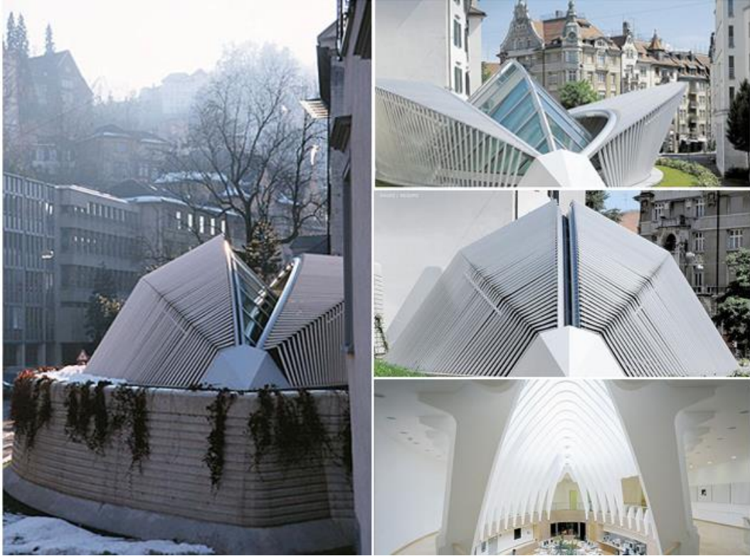
Resim 3.86. Santiago Calatrava, Emergency Services Centre , Saint Gallen, Switzerland, 1998 [ http://www.calatrava.com ]
