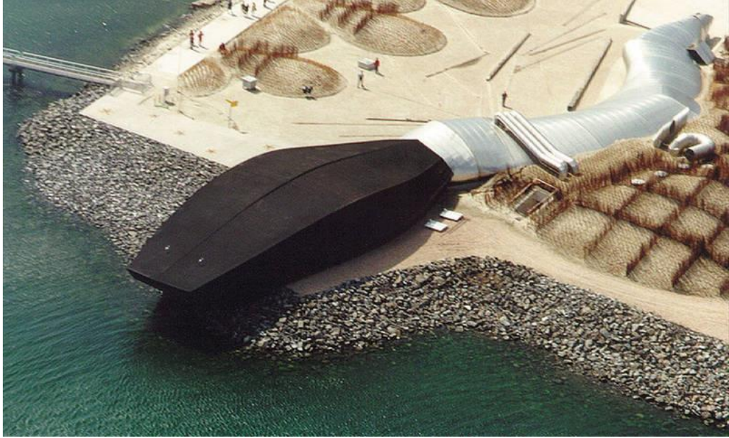
Resim 3.53. Kas Oosterhuis –Tuzlu Su Pavyonu( Saltwater Pavilion ), 1997, Lars Spuybroek –Taze Su Pavyonu( Freshwater Pavilion ), 1997[Oosterhuis, 1997]
