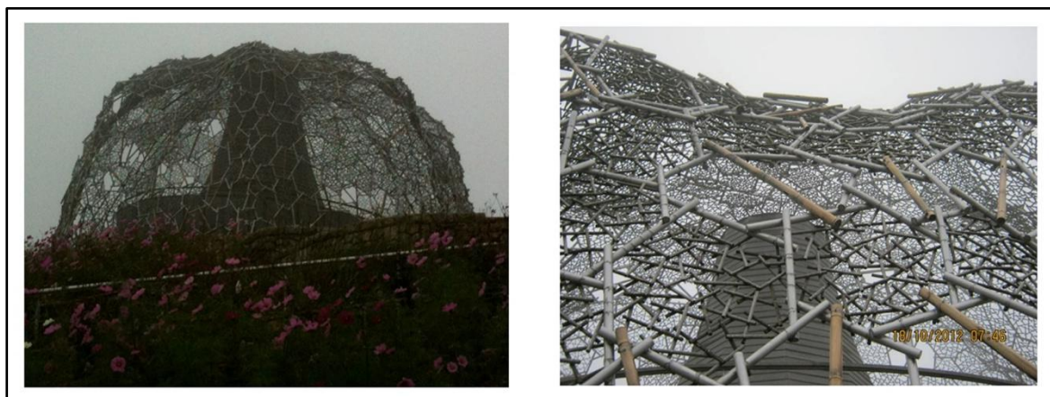
Figure 3.18. Mount Rokko-Shidare Observatory RF structure façade (Popovic Larsen, 2014).
