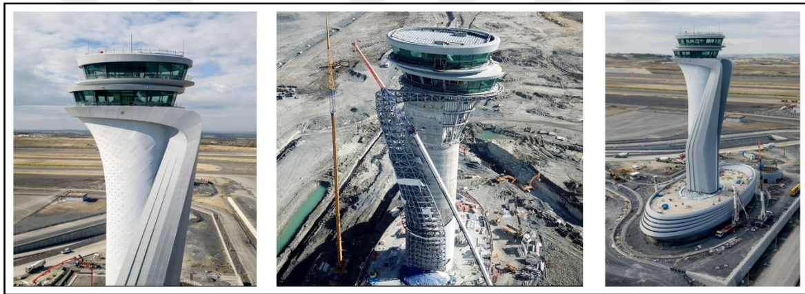
Figure 4.5. İstanbul ATC Tower views (Metalyapı, 2013).
