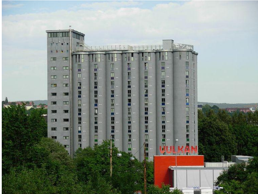
Şekil 4.48. Grünerlokka Studenthus / Yeni cephe ( https://inhabitat.com/oslos-grunerlokka-studenthus-is-a-student-housing-complex-located-in-a-former-grain-elevator/ )
