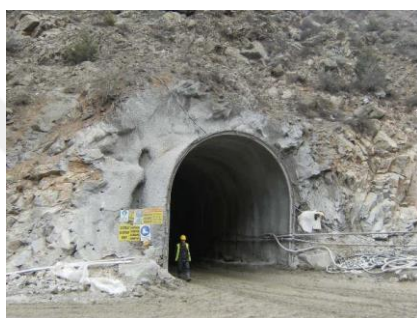
Approach tunnel, photo by Zafer Durmaz (2009)
