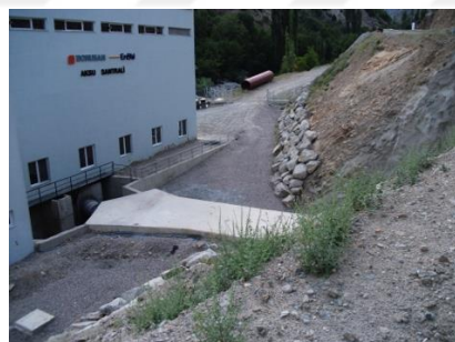
Borusan Aksu Plant
