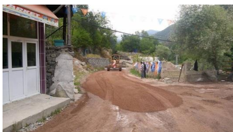
Road construction, 2015 (Photo by Hanifi Aksu)
