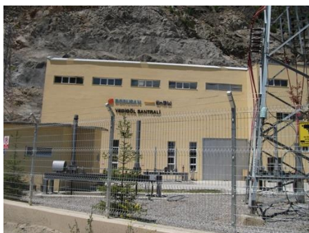
Borusan Yedigöl Plant
