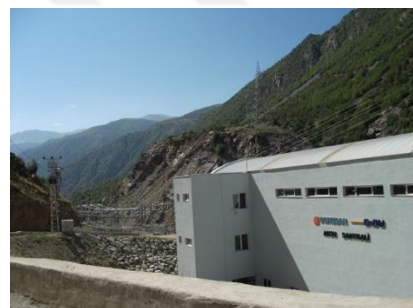
Borusan Aksu Plant
