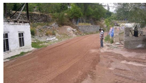
Road construction, 2015 (Photo by Hanifi Aksu)
