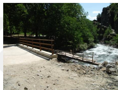
The bridge built by Borusan
