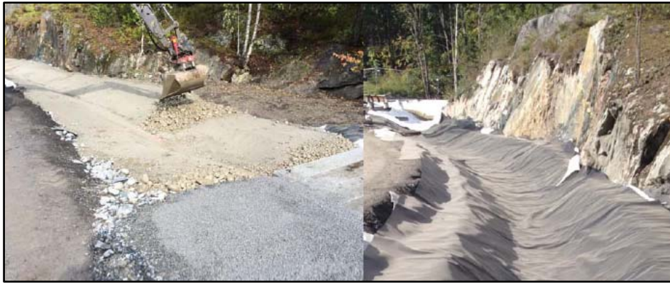
Figure 3.13. Construction of streambed for providing infiltration function, Julsberg Stream Project. [Source: Rapp, O. (2019)]
