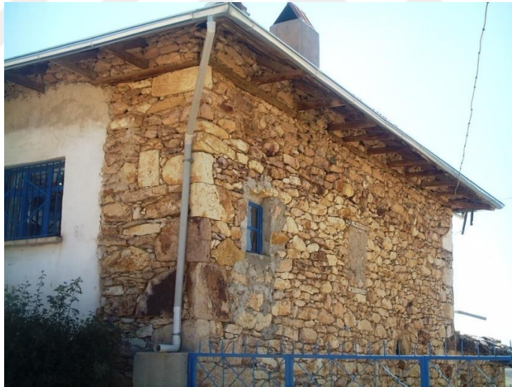
Figure 4.4 Mud mortared rubble stone building in Gümüşkol Village (Bilgin et al., 2015)
