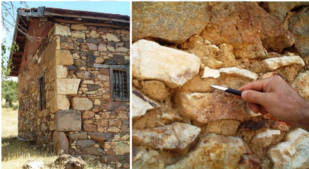
Figure 4.5 a) Mud mortared building in Katrancılar village constructed in 1945, b) A close view of the rubble stone and mud mortar wall (Bilgin et al., 2015).
