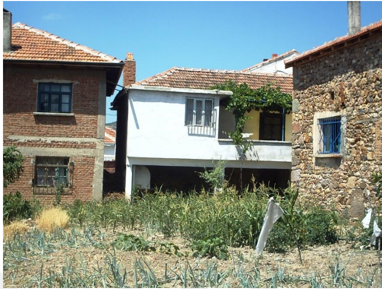
Figure 4.6 Various structure types: mud mortared rubble stone building on the right, lime mortared brick walls and reinforced concrete structures in the middle and on the left (Bilgin et al., 2015).
