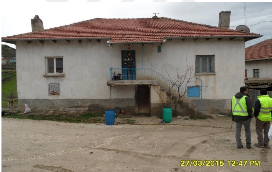
Figure 4.7 Two-story, mud mortared rubble stone building belonging to Sami Yıldırım (Bilgin et al., 2015)
