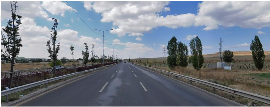
Figure 27. Transportation lines restricting accessibility of the Atatürk Forest Farm
