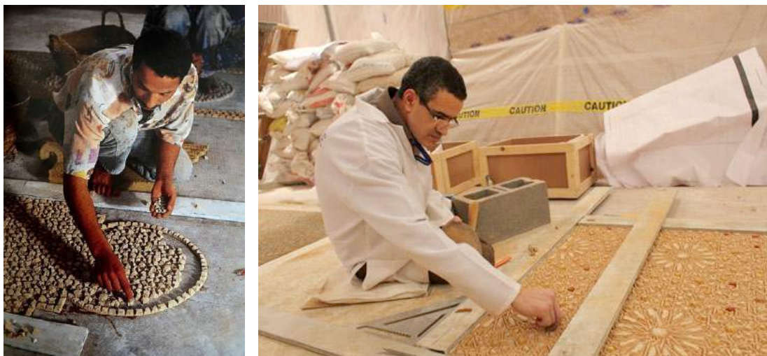
Figure 3.13 : Zellij craftsmen execute reverse assemblage to form larger plates (Photos, left: Castera (1999) and right: Fremson (2011)).
