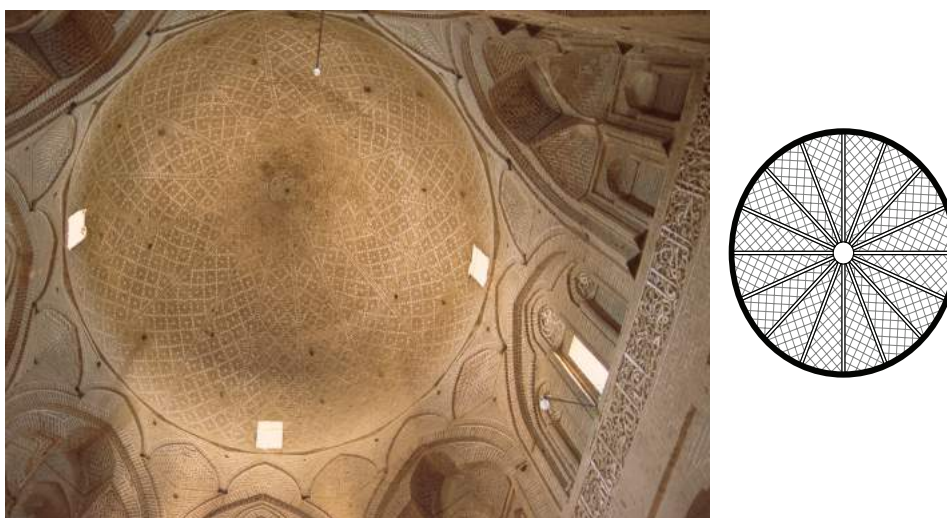
Figure 5.50 : The domical façade decoration of Masjid-i Jami' of Ardistan based on a sixteen fold vertical segmentation (Left: image from “Aga Khan Visual Archive,” 2017).
