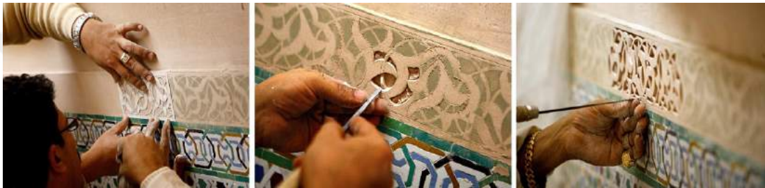
Figure 4.8 : Prior to carving, the pattern is drawn onto the gypsum surface by using a template (Photos from Fremson (2011)).
