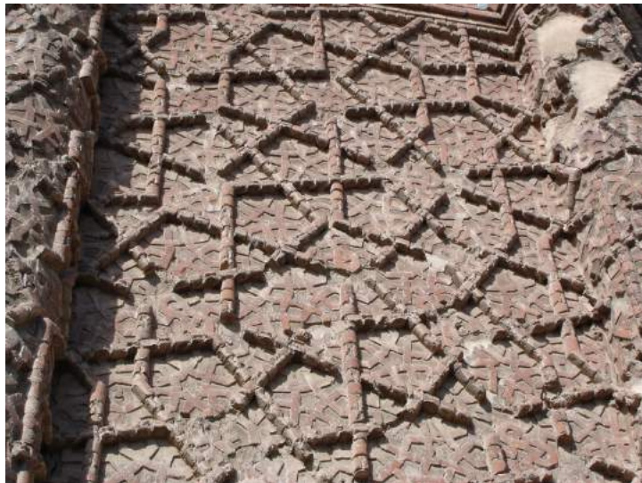
Figure 5.28 : Close ups of the dual level design in Gunbad-i Qabud in Maraga, Iran (1196-97 A.D). (Photos from Mortel (2005) and Archnet (2018)).
