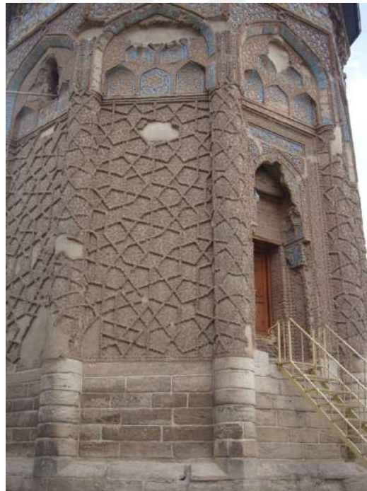
Figure 5.29 : Individual modules for the column curvature Gunbad-i Qabud in Maraga, Iran (1196-97 A.D). (Photo Archnet (2018)).
