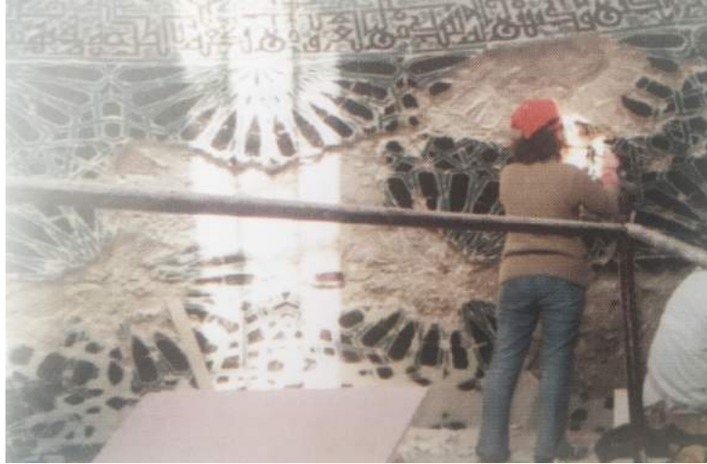
Figure 5.77 : A restaurateur working on the dome surface (Erdemir, 2001, p. 176).
