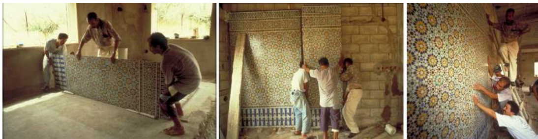
Figure 5.4 : Moroccan craftsmen installing rectangular cut tile panels (Images Sanders (n.d.)).
