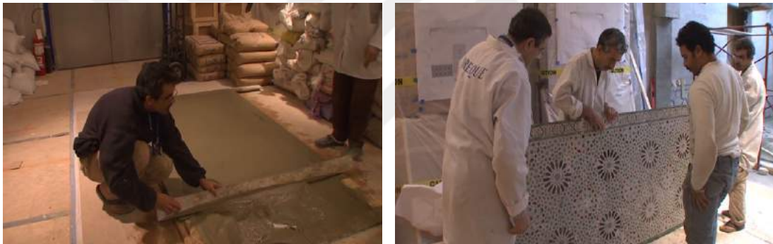
Figure 3.15 : Ones the mortar is poured, a larger cut tile panel is obtained (Campbell, 2011).
