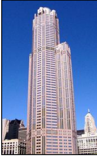
Şekil 2.13 311 South Wacker Drive
