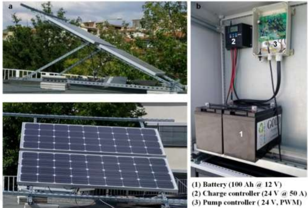
Figure 5.7 Energy system for prototype I
