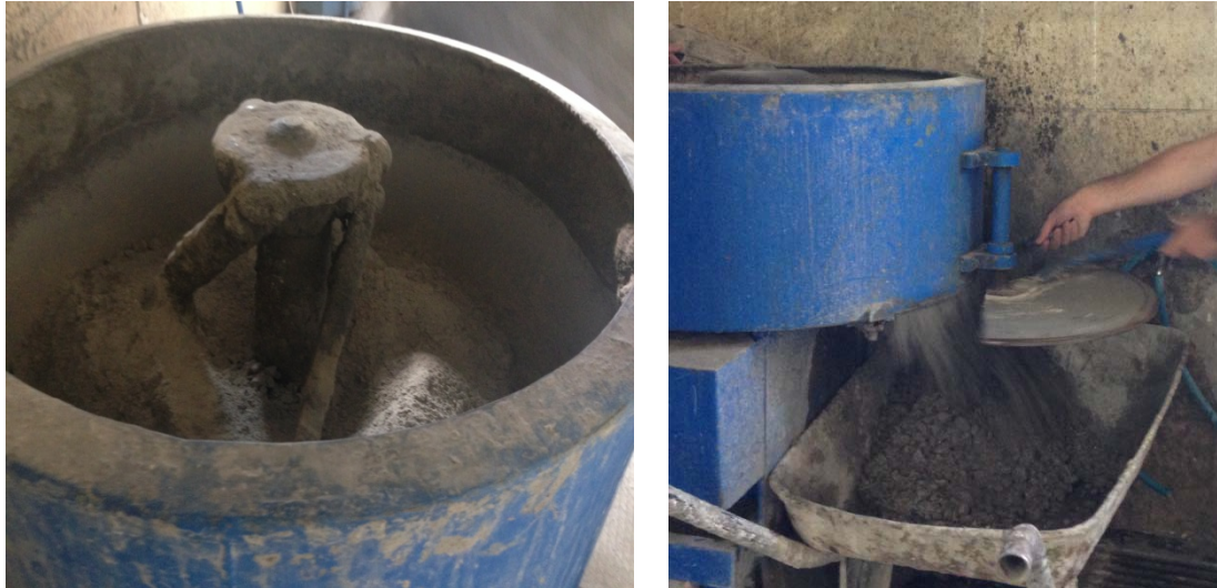
Figure 3.3 Concrete mixing in concrete mixing machine
