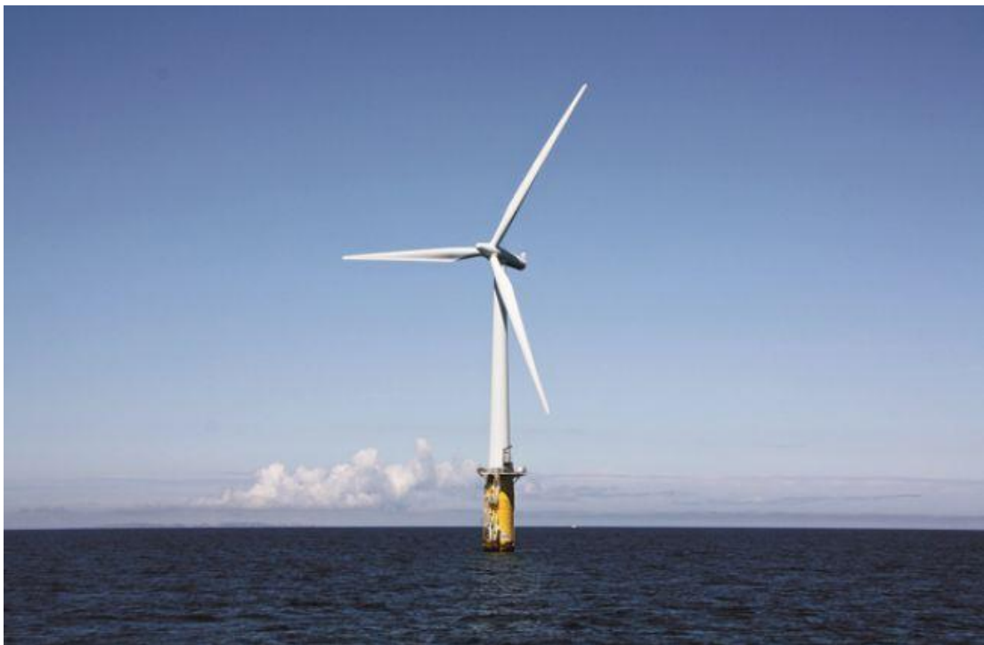
Figure 2.4 : An offshore wind turbine.
