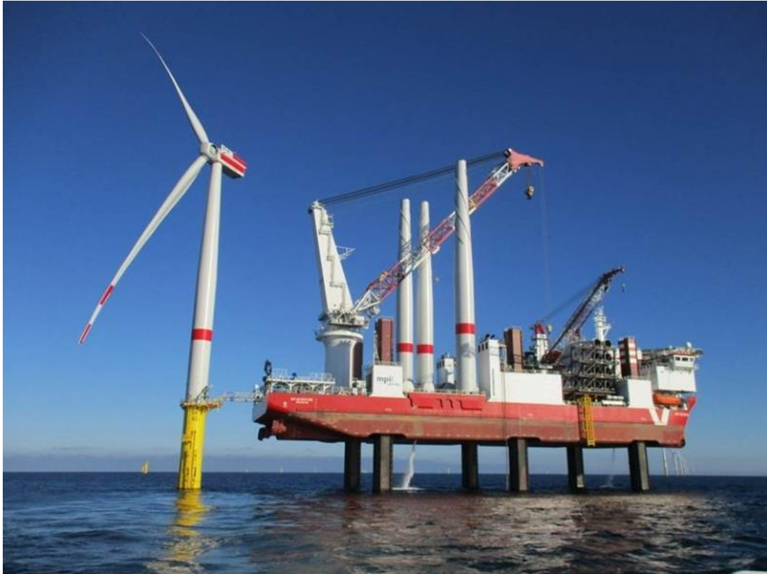
Figure 3.2 : Wind turbine installation site.
