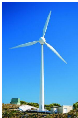
Figure 2.3 : A modern wind turbine.
