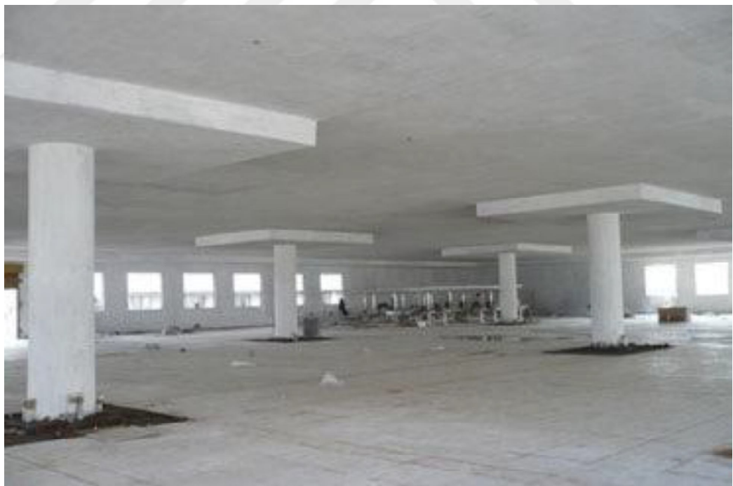
Figure 3.4. Drop Panel in Flat Slab
