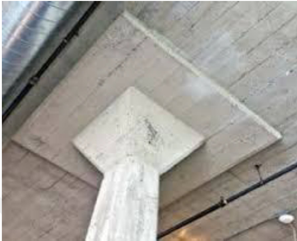
Figure 3.5. Column head in flat slab
