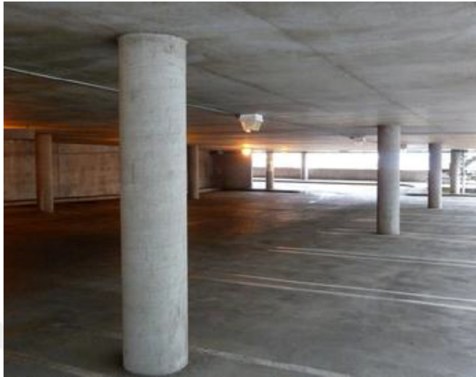
Figure 3.2. Flat Flooring System
