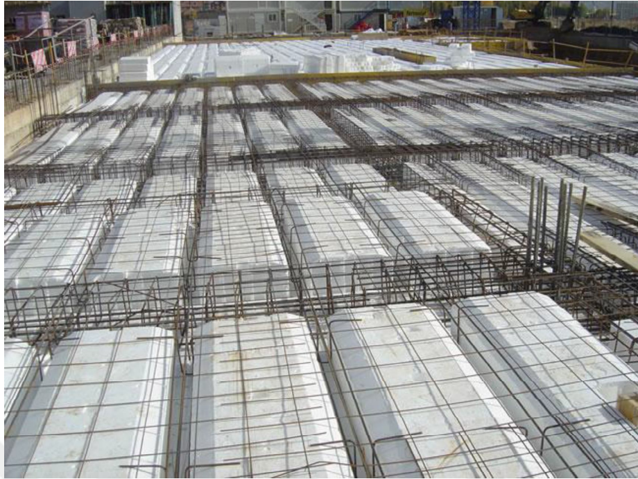
Figure 3.6. Ribbed flooring system in one way direction
