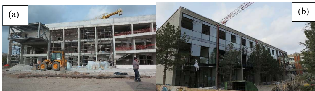
Figure 74 Images of under construction (a) Educational Science Department Building, (b) Classroom Hall Building.
