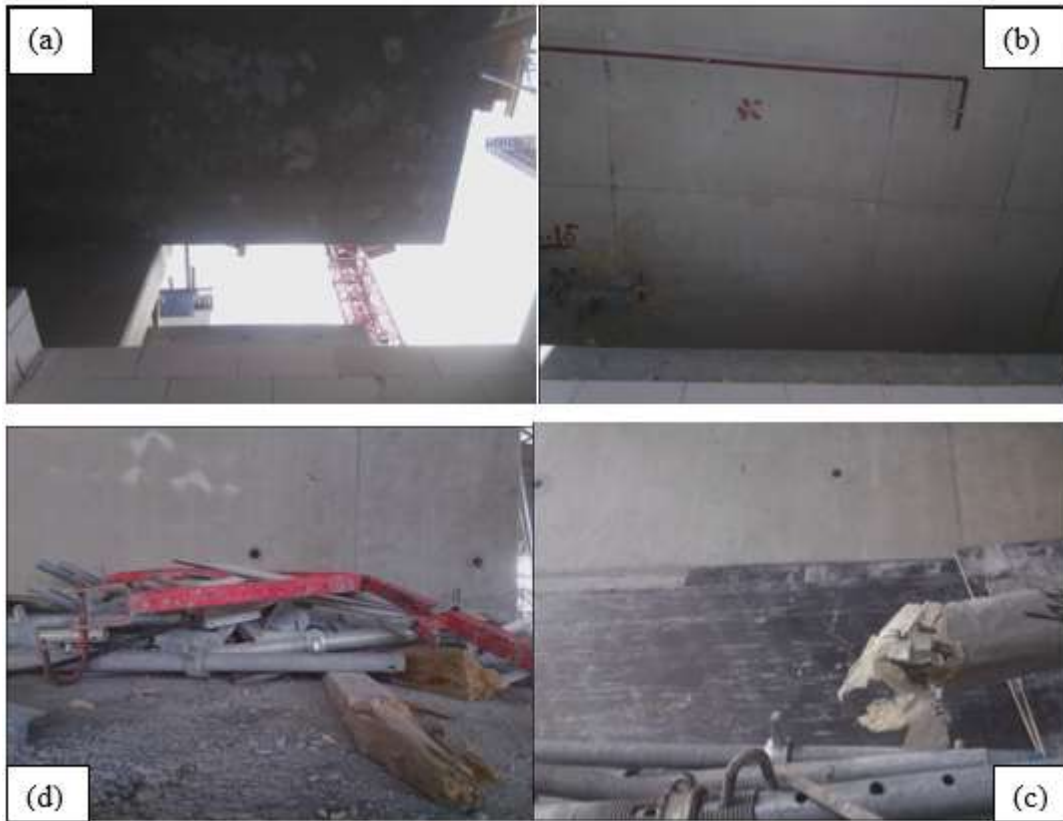
Figure 51 Poor Image Examples (a)-(b) Acquired at 30% misses EOI and captures roof slab, (c)-(d) Images acquired at 90% captures clutter on the floor next to wall.
