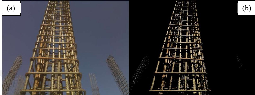
Figure 83 (a) Image with reinforcement (b) Extracted reinforcement from image.
