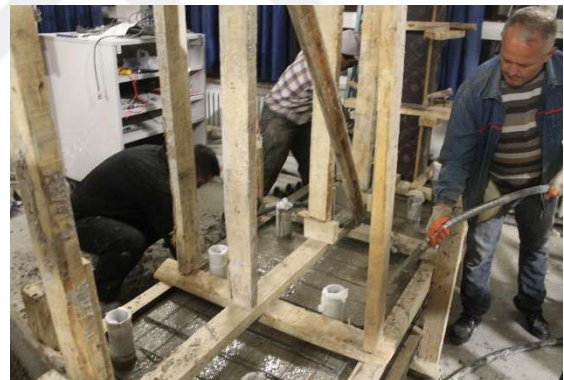
(b) Vibration process of concrete
