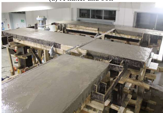
(c) Finished-surface of slabs
