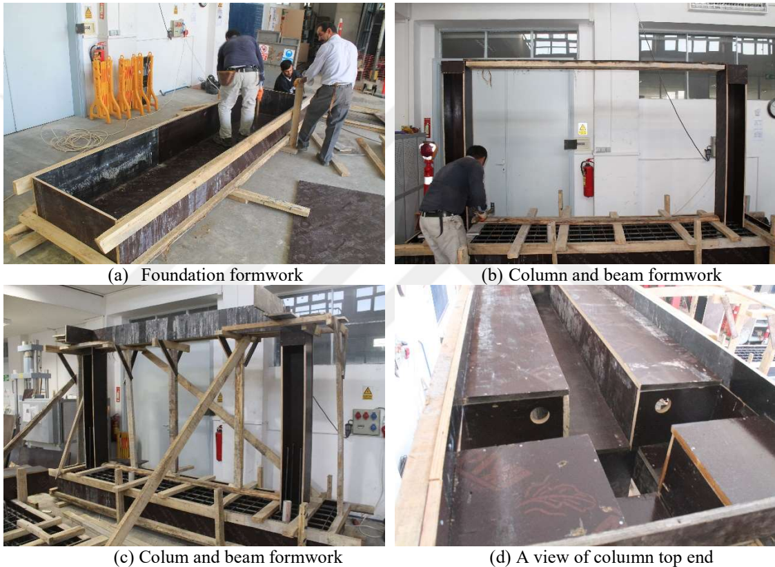
Figure 3.26. Formwork works
