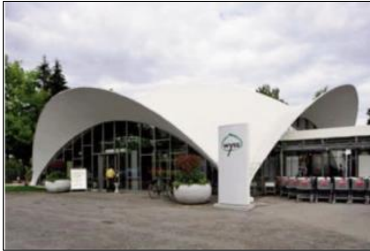
Figure 2.8: Concrete shell of Wyss Garden Centre by Heinz Isler
