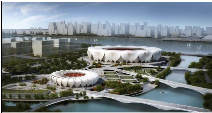
Figure 2.20: The Olympic Stadium and the Tennis Center in Hangzhou
