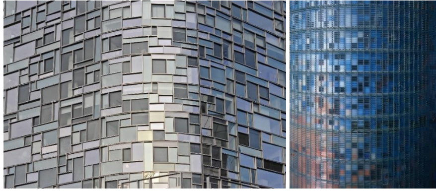
Figure 2.15 : Examples for parametric facade design, 100 Eleventh Avenue (on the left), Torre Agbar (on the right), both by Jean Nouvel (Url-10).
