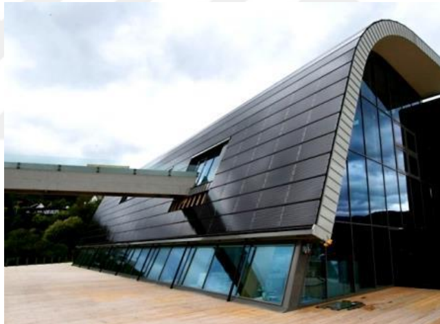
Figure 2.10 : Physical and visual integration of facade with roof system (Oseana Art and Culture Center, Bergen, Norway, Url-6).
