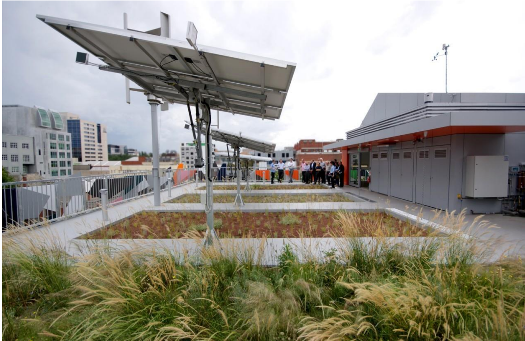
Figure 4.22. Green roof and solar panels (Studio 505, n.d.)
