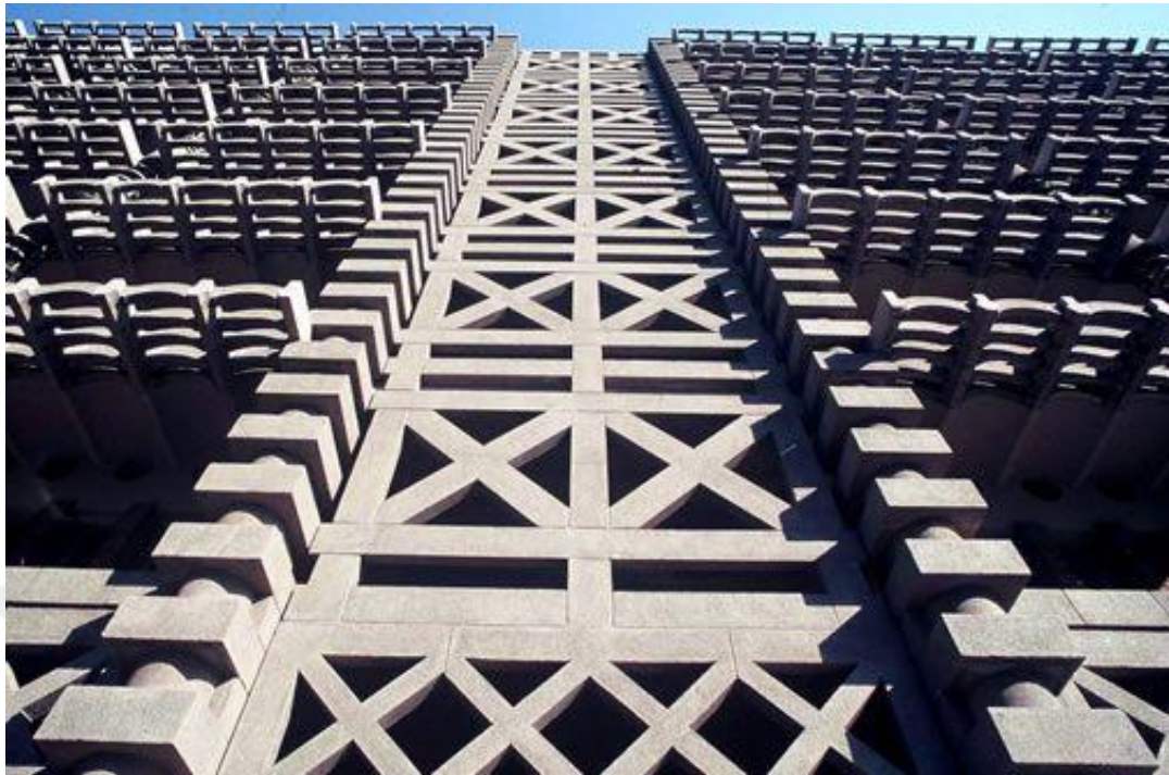
Figure 4.11. Facade detail (Tunguz, 2016)
