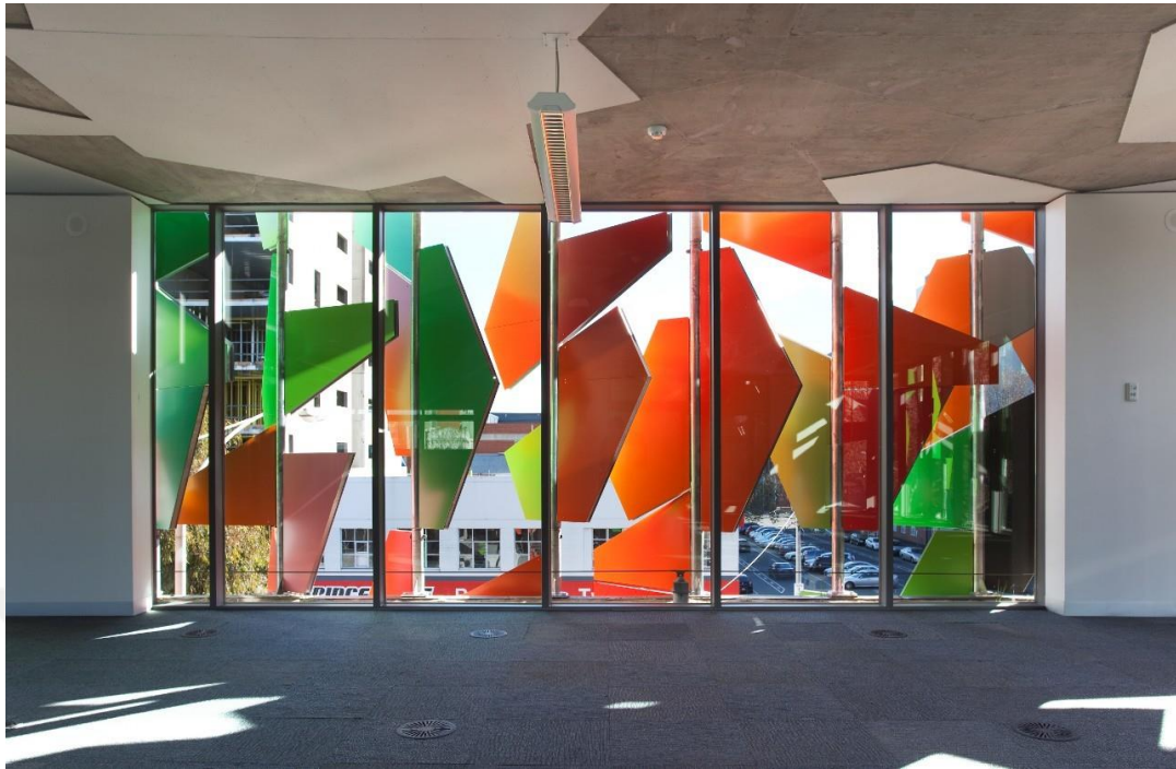
Figure 4.24. Shading and glaring prevention seen from inside (Hosking, n.d.)
