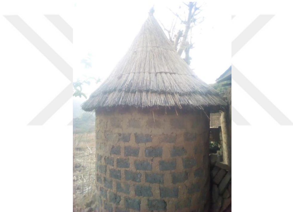
Plate 5: Photography of a thatch roof in a typical Sokoto vernacular architecture building (Ibrahim, 2023)
