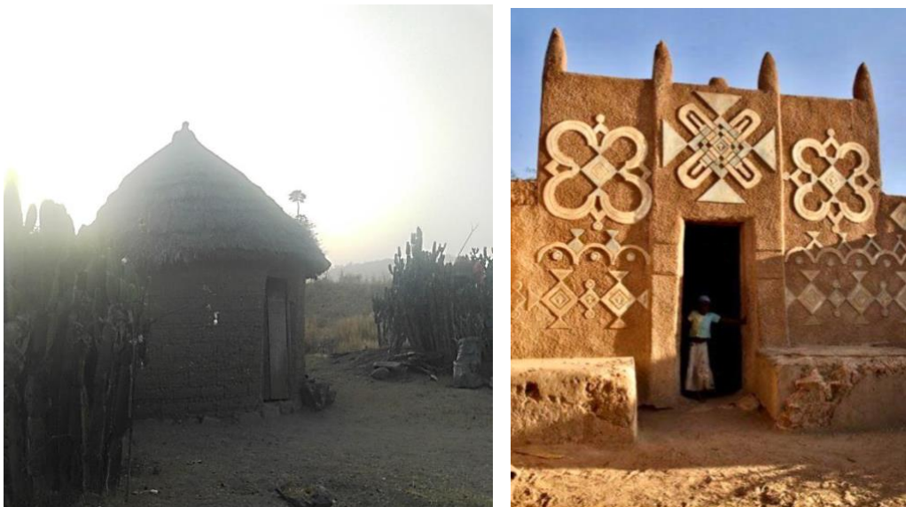
Plate 8: Photograph of a recent traditional circular and rectangular vernacular building typology in Sokoto State (Ibrahim, 2023)
