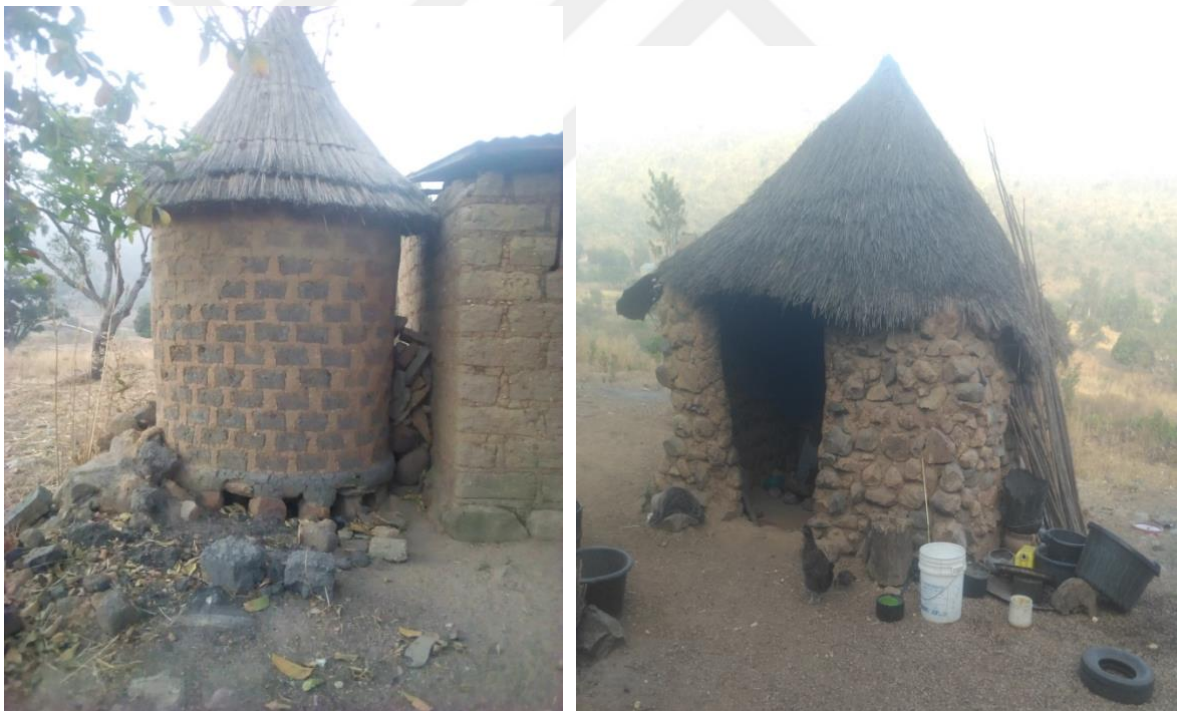
Plate 4: Photography of Stones used for foundations and wall construction in a traditional building in Sokoto State, Nigeria (Ibrahim, 2023)
