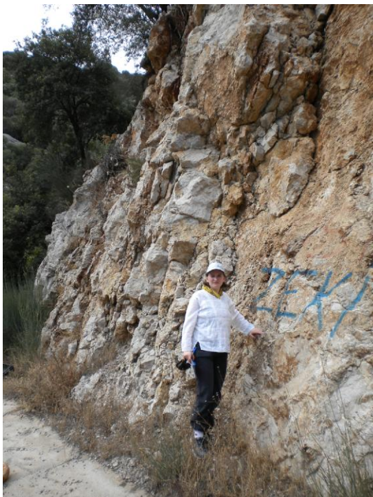
Figure 4.5. Photograph showing main discontinuities developed in the limestone at Km: 25+900.
