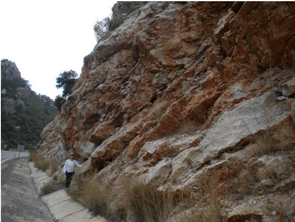
Figure 3.12. A view from the limestone facing north at Km: 25+900.
