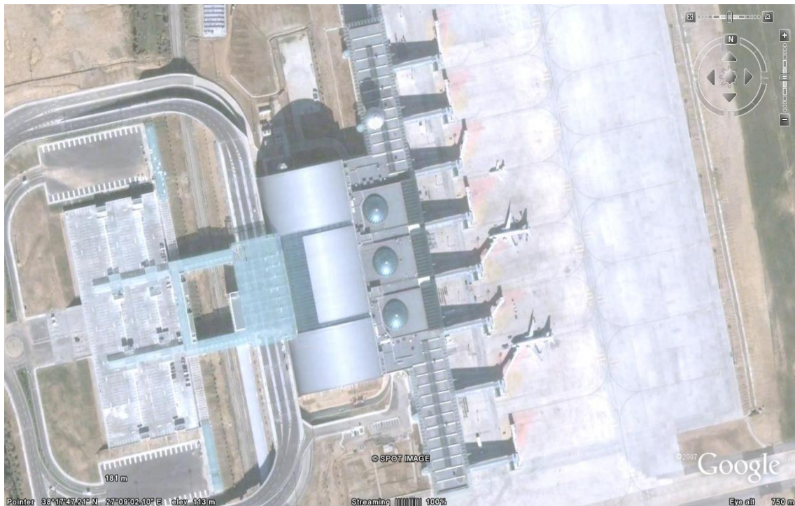
Figure 2.1. ADM Building Birds Eye View from Google-Earth.
