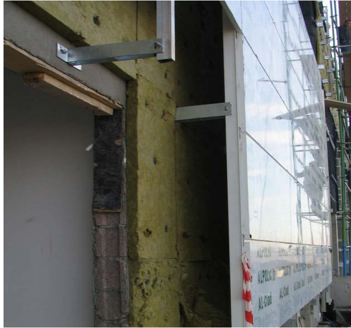
Figure 3.11. External Wall of ADM Building.
