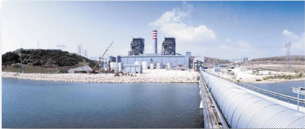
Figure 33: Iskenderun Power Plant [5]
