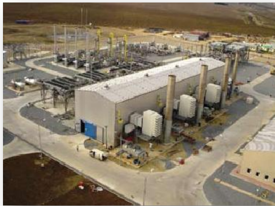
Figure 31: Silivri Natural Gas Storage Facilities [29]
