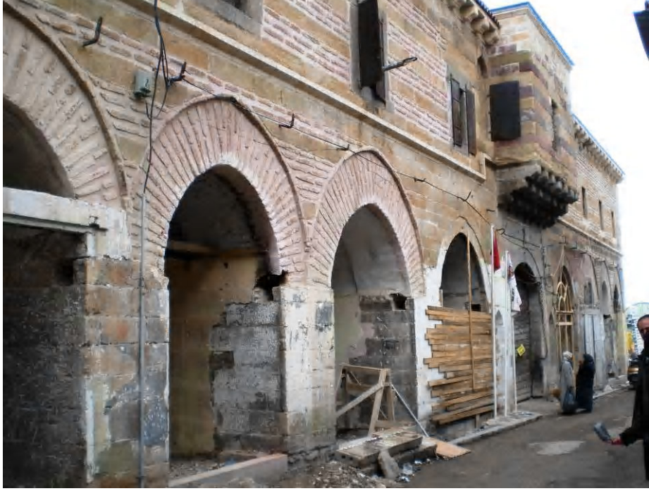
Fot.2. 2.182. Merzifon Taşhan Güney Cephesi (V.G.M.A.)
