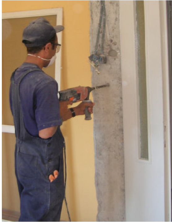
Figure 3.5 Drilling of the holes
