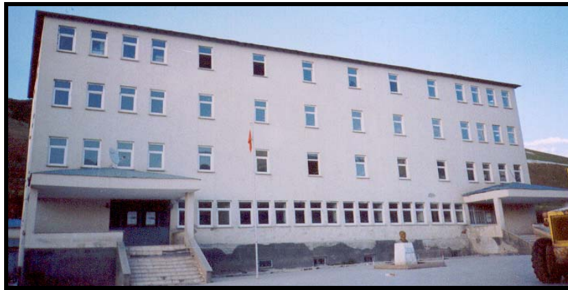
Figure 5.1 Front View of the School Building
