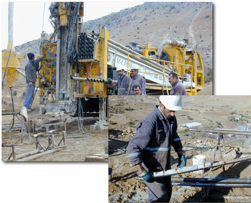
Figure 3.1 Acid Mine Drainage Core Sampling
