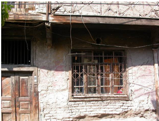
Figure 2.4 General view of Öksüzler Lane House
