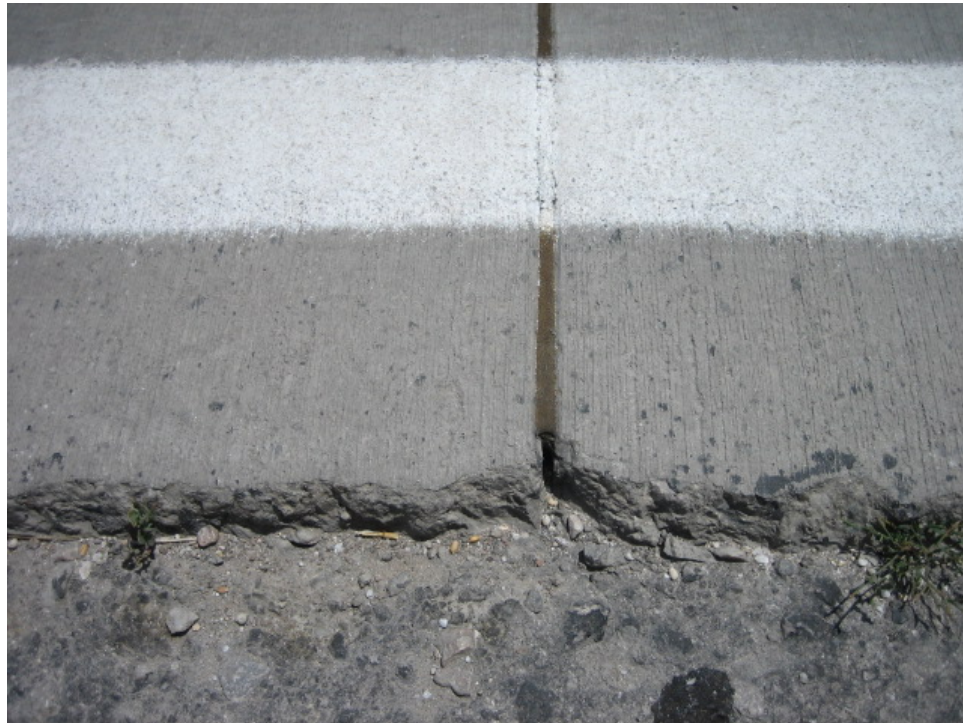
Figure 2.15 A photograph taken at September 2006 shows that the status of the joints and of the sealing material in between is still in good condition
