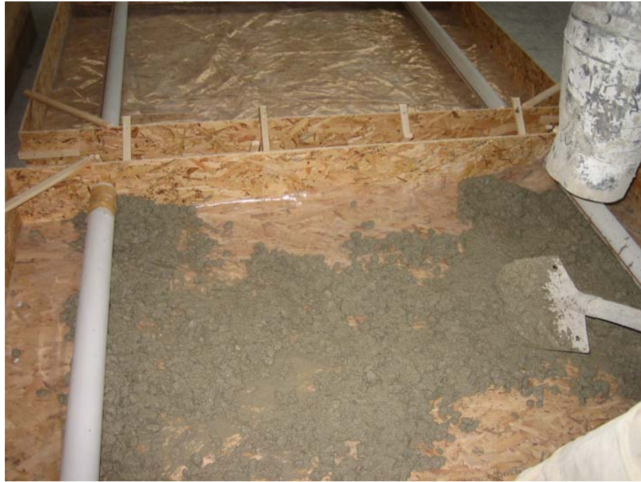
Figure 3.3 Final status of forms while placement of concrete has just begun
