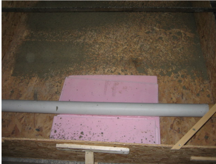
Figure 3.4 Two pieces of foam board being tucked under the pipe for the purpose of leaving a void at known depth
