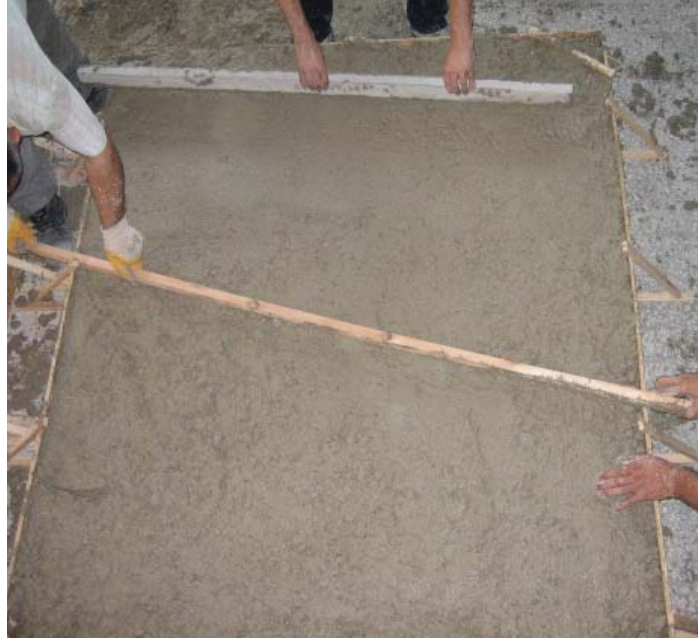
Figure 3.5 Smoothing the surface of one of the slabs
